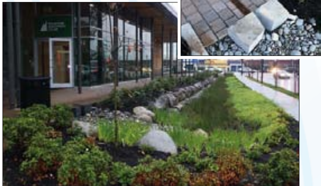
The Mountain Equipment Co-op store rain garden in North Vancouver, BC.
